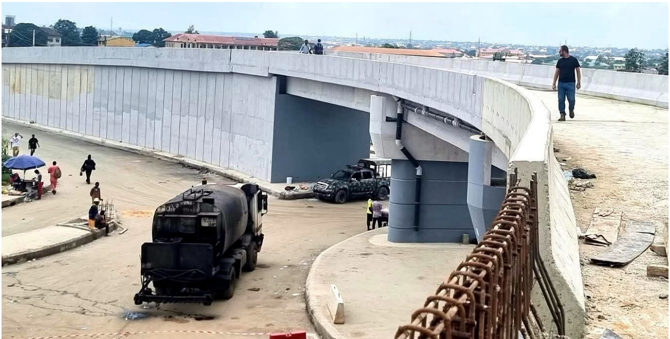
Control post interchange Flyover Owerri
