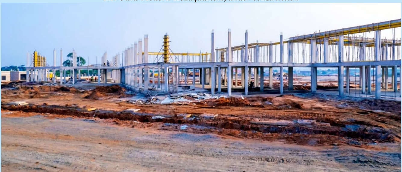
Construction of Imo digital bus terminal
