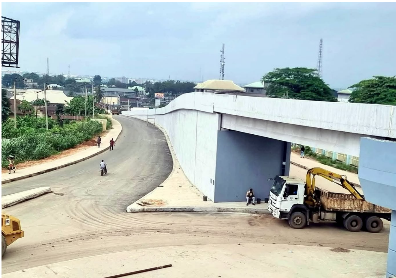
Control post interchange Flyover Owerri
