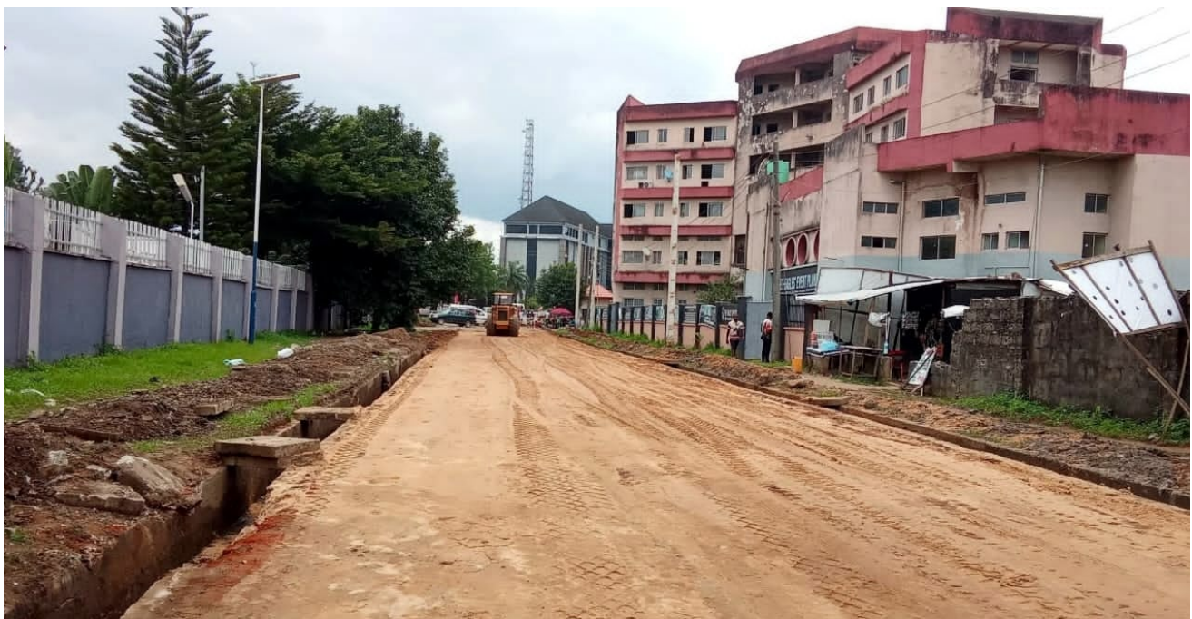
Owerri Ph Road, drainage construction
