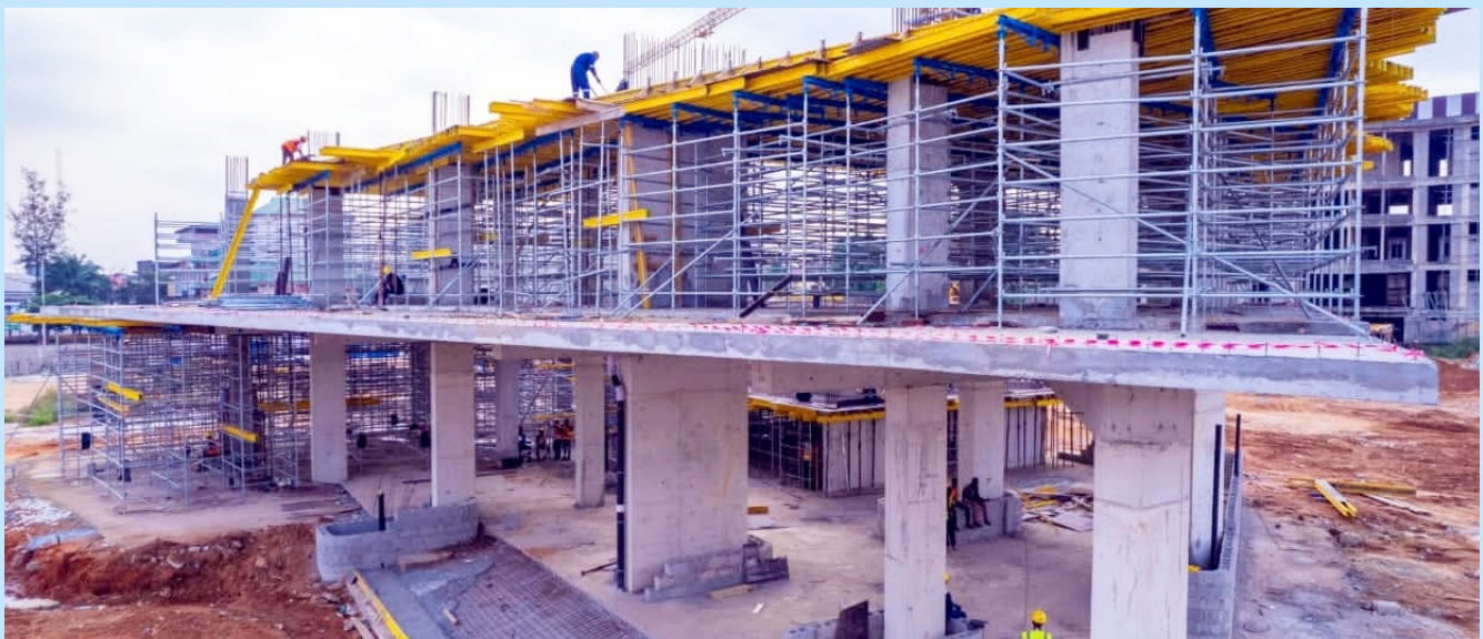
IIR Ultra-Modern Headquarters, under construction
