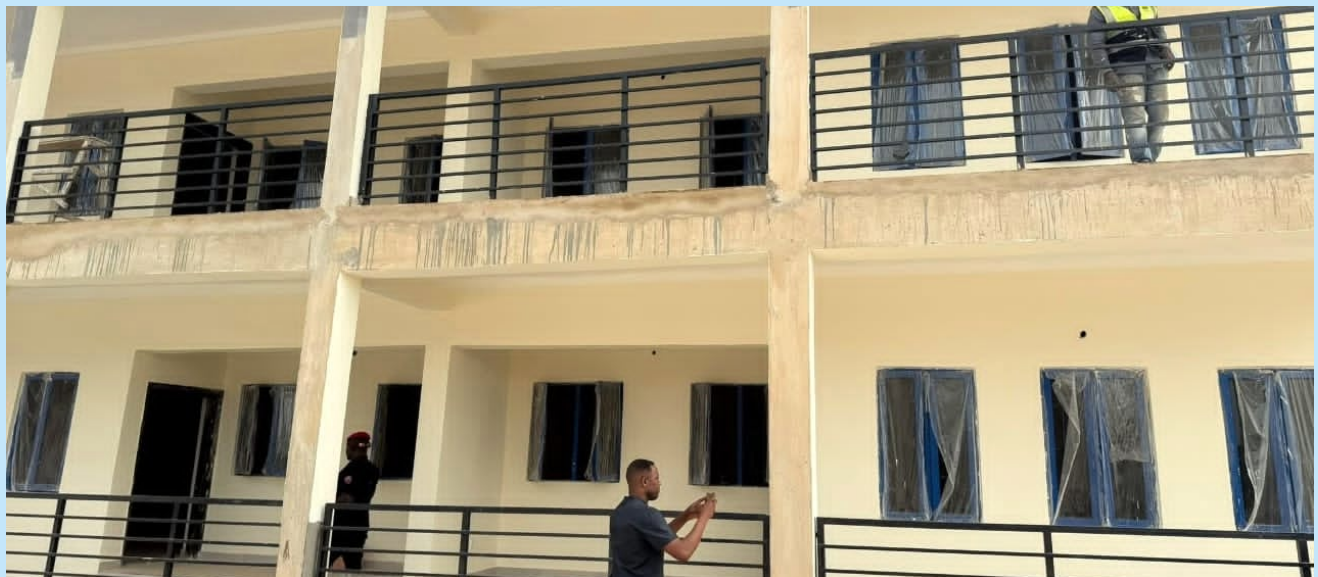
Constriction of New Airforce building, Airport Road
