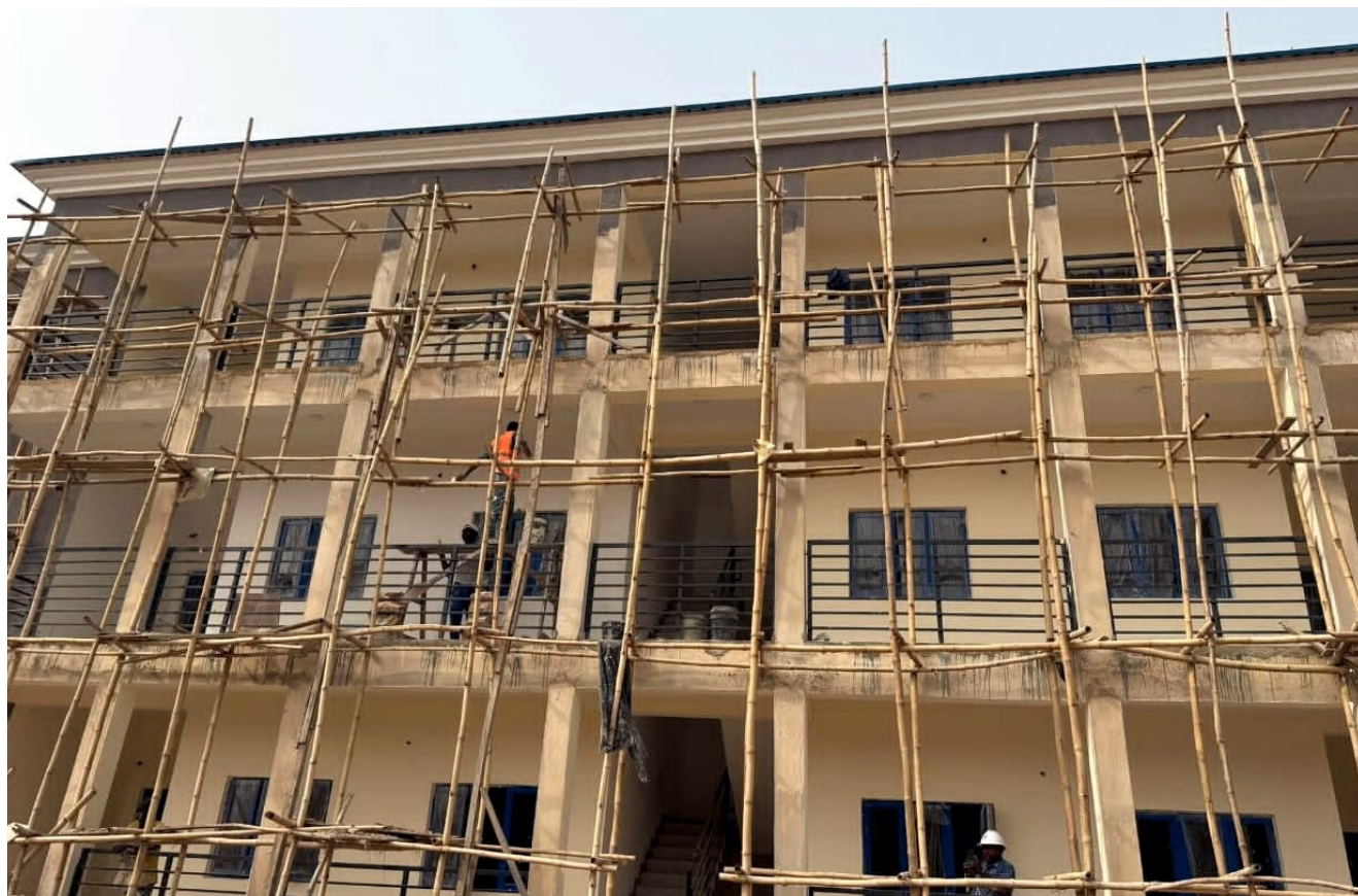
Construction of New Airforce Building, Airport Road
