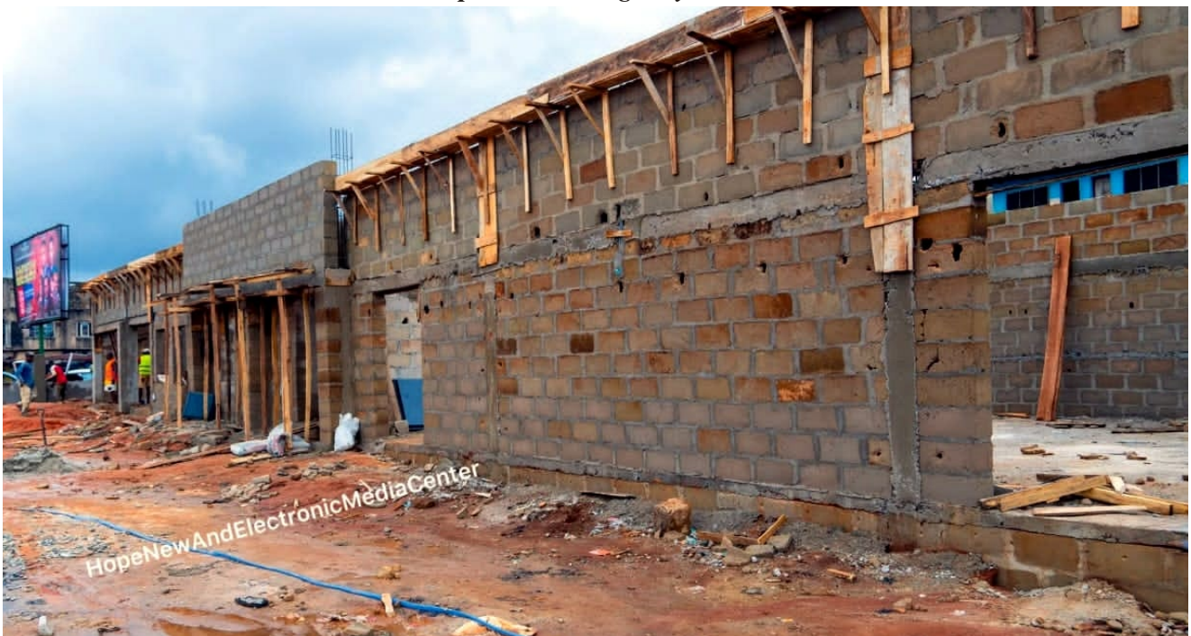
Construction of Tech Hub Computer Village Owerri
