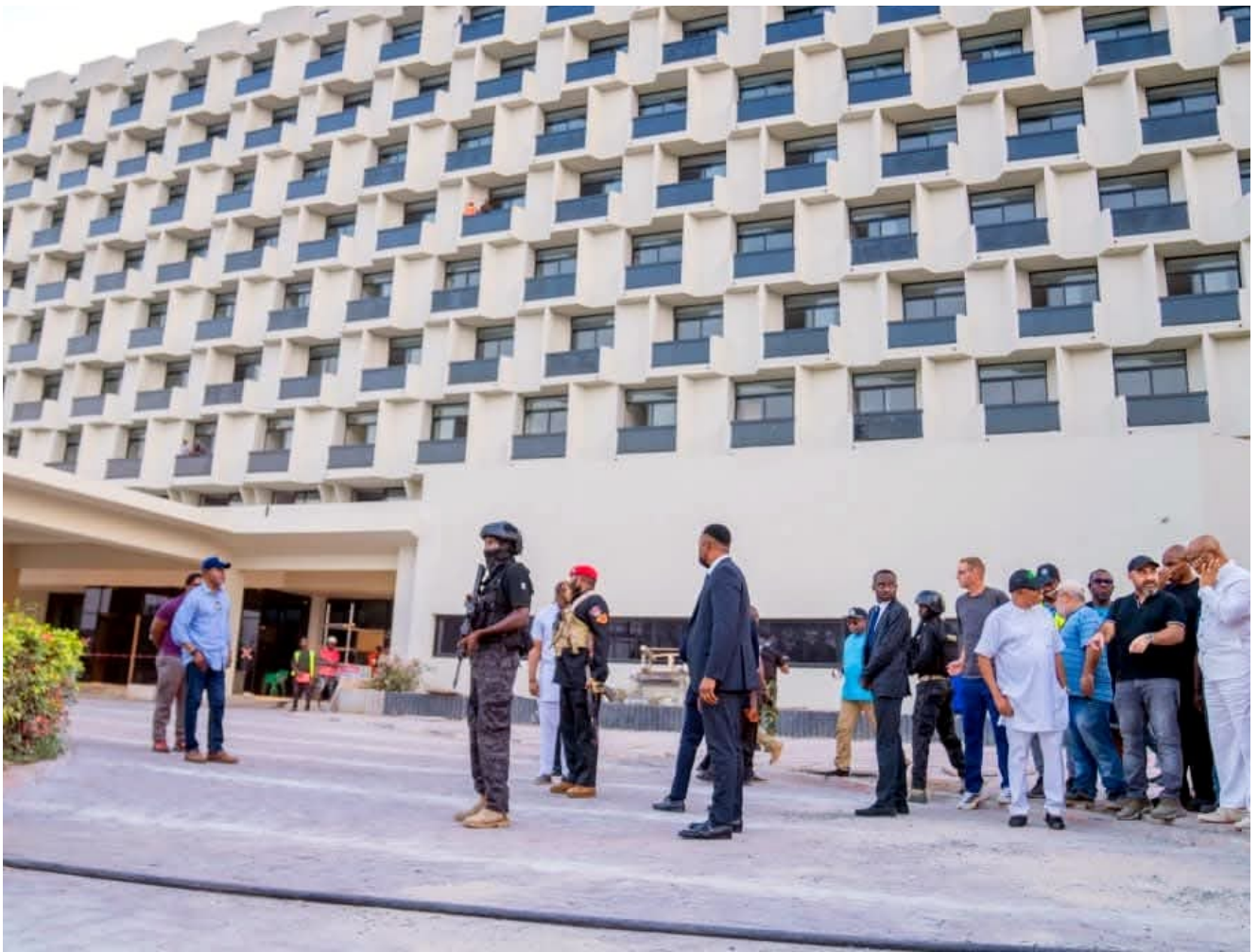
Rehabilitated New Imo Concorde Hotel
